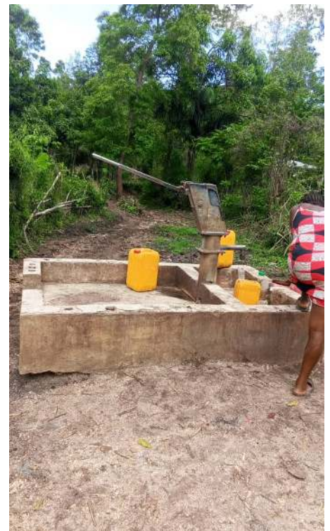
Fig. 5 — Functional pump currently in use
