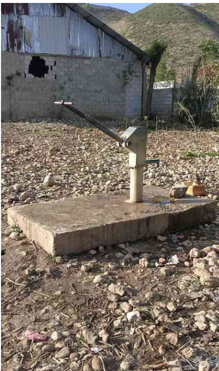
Fig. 3 — Pump installed on rocky ground, illustrating the constraints of site placement
