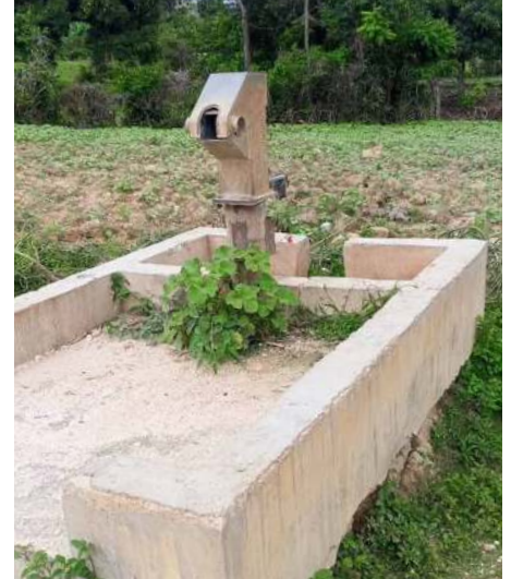
Fig. 2 — Non-functional community pump, overtaken by vegetation
